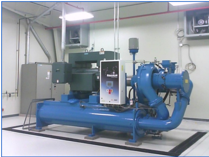
F.S.Elliott P700 1,500 Horsepower Centrifugal Compressor System
